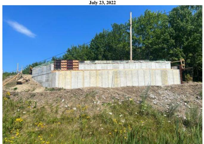
Looking at the western abutment. Crews have made progress rehabilitating the existing abutment for the new bridge girders to be placed
