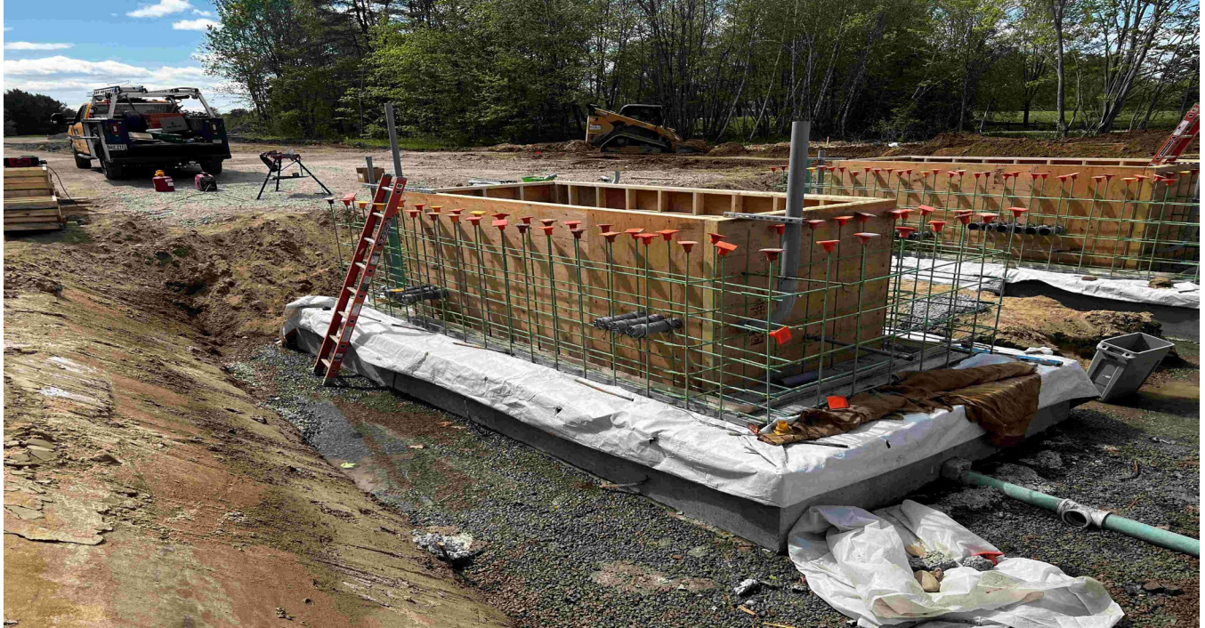
The north bound entering toll booth foundation formwork are coming along.
