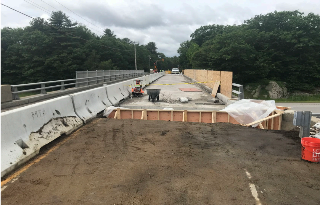
Mountain Road Looking West showing recent concrete repairs.
