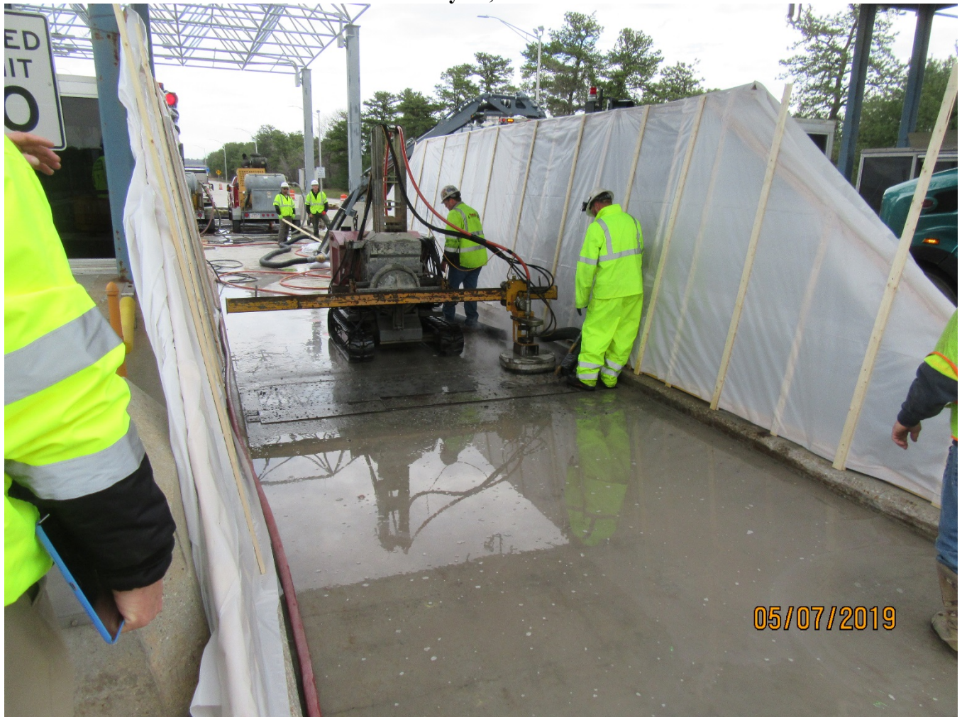
Hydro-blasting concrete slab at New Gloucester
