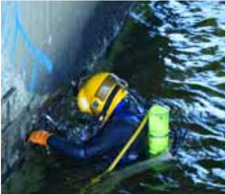
Specially trained scuba diving construction workers were required to perform rehabilitation of the Cobbosseecontee Stream bridge in West Gardiner.
