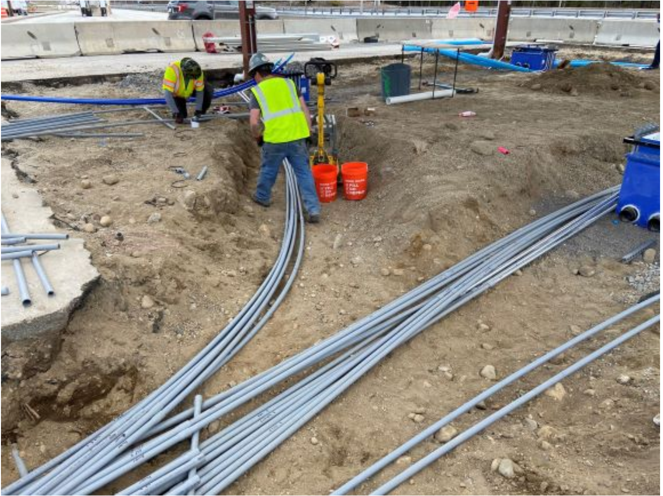
SRS crew installs electrical conduits for the new gas fueling system.
