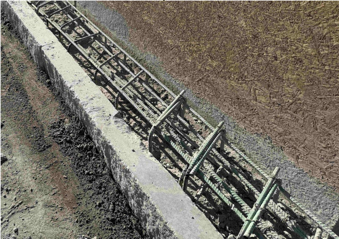
Looking south at the southbound bridge curb with the reinforcing steel showing
