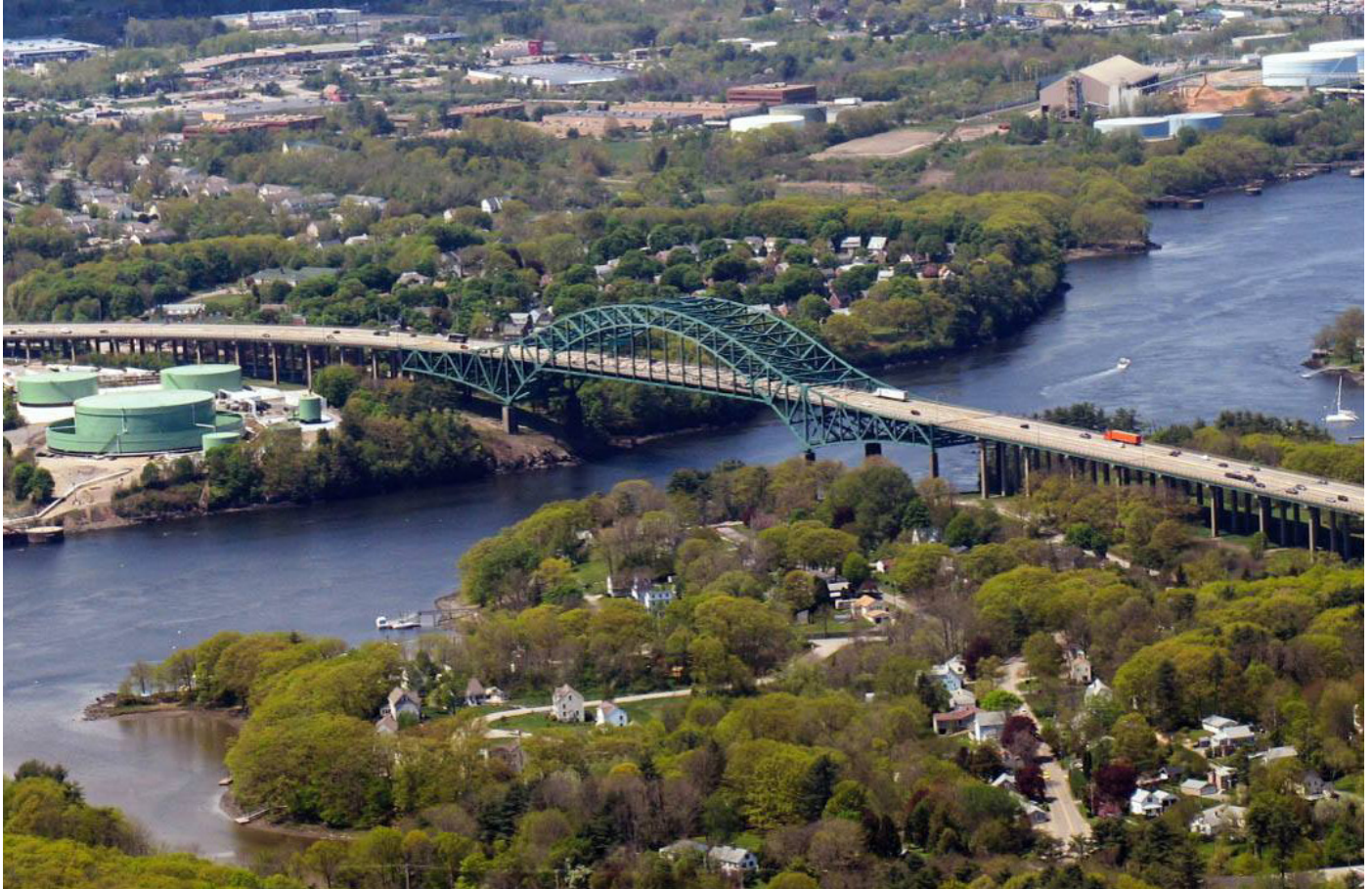
PHOTO 27: PISCATAQUA RIVER BRIDGE
