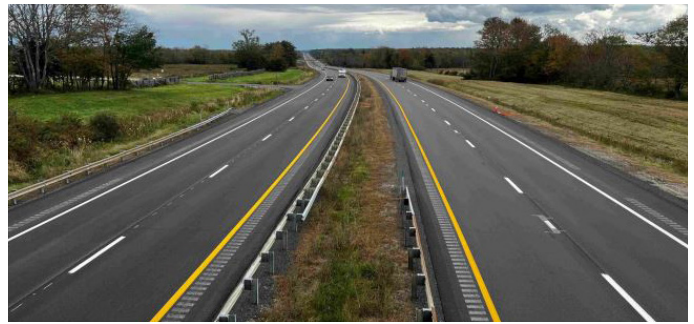
PHOTO 5: ROADWAY MARKINGS MILE 88
