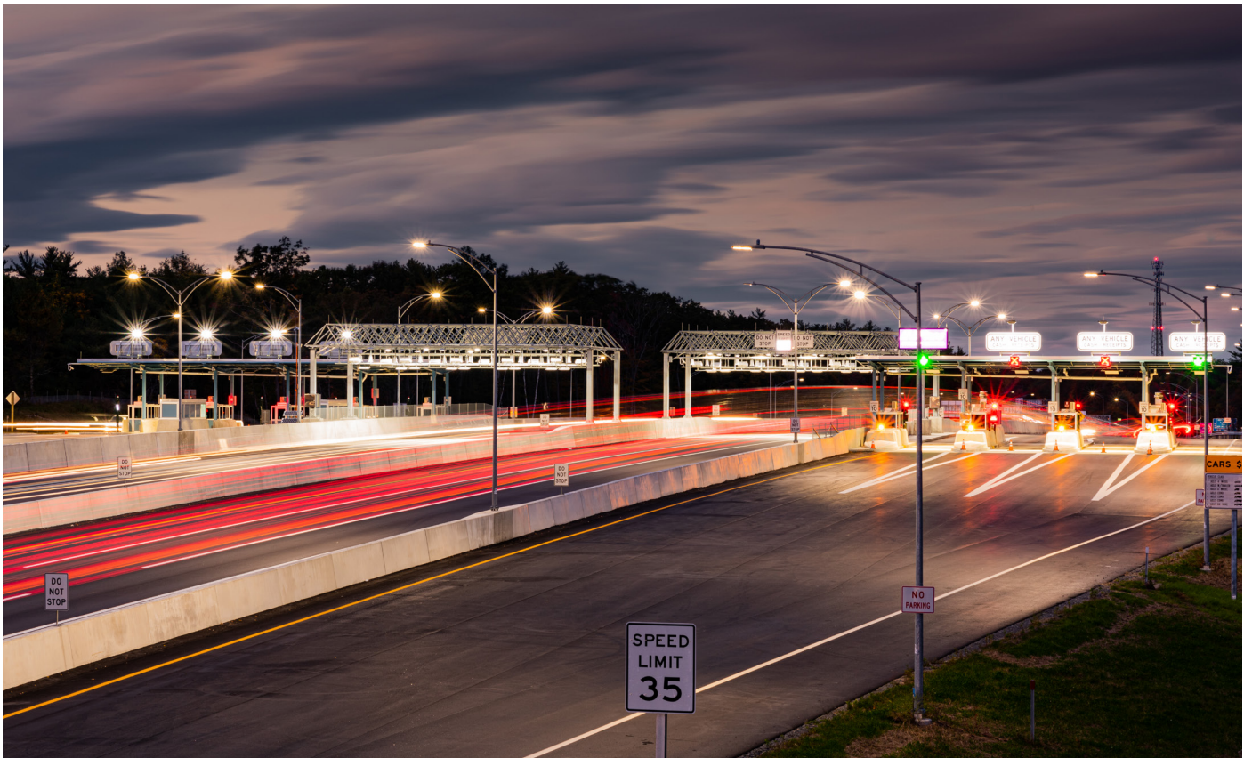
PHOTO 21: YORK TOLL PLAZA
