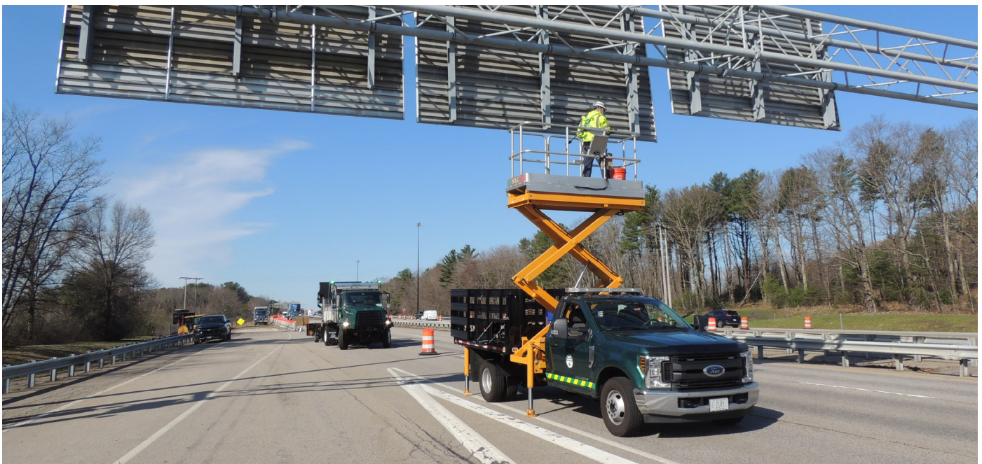
PHOTO 20: OVERHEAD SIGN BRIDGE INSPECTION
