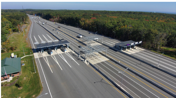
PHOTO 8: YORK TOLL PLAZA
