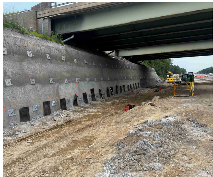
PHOTO 17: SACO INTERCHANGE BRIDGE MODIFICATIONS
