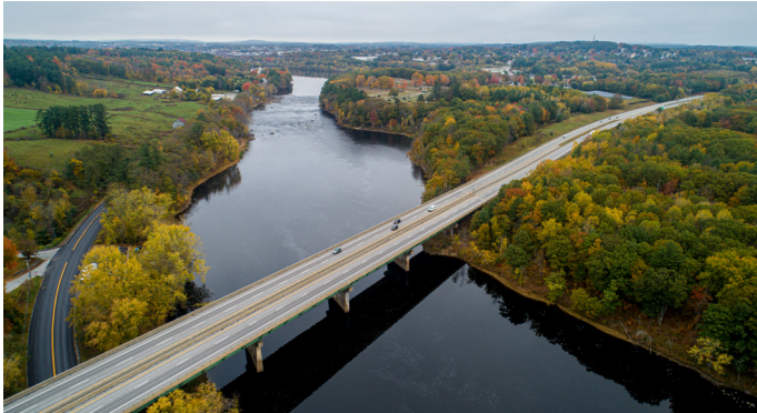
PHOTO 14: ANDROSCOGGIN RIVER BRIDGES
