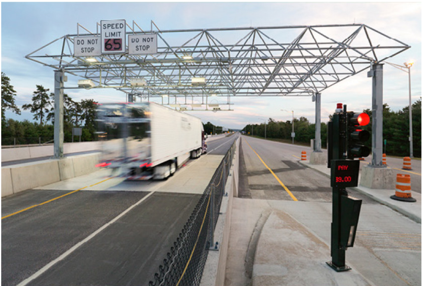
PHOTO 22: NEW GLOUCESTER TOLL PLAZA
