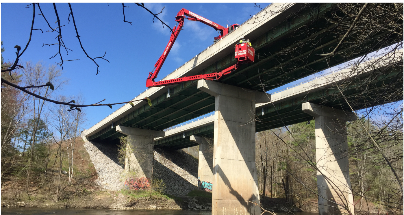
PHOTO 1: PRESUMPCOT RIVER FALMOUTH SPUR BRIDGE INSPECTION
