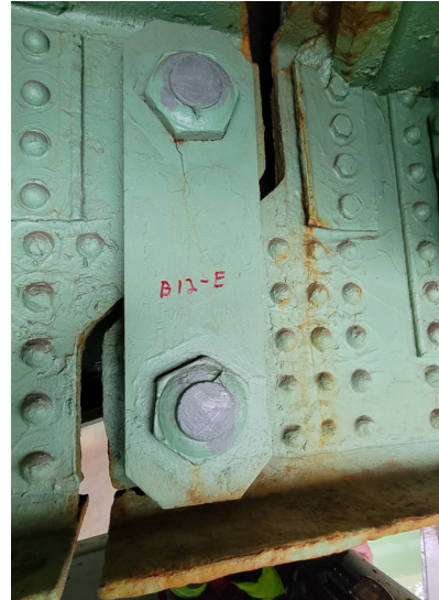
PHOTO 16: YORK RIVER BRIDGES PIN-AND-LINK CONNECTION
