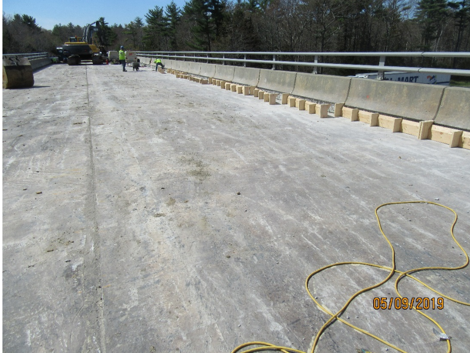
North Berwick Road Looking West laying out formwork
