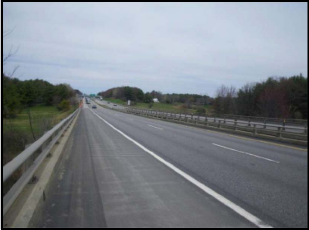
Figure 2 - Southbound Bridge Top of Deck, Looking North
