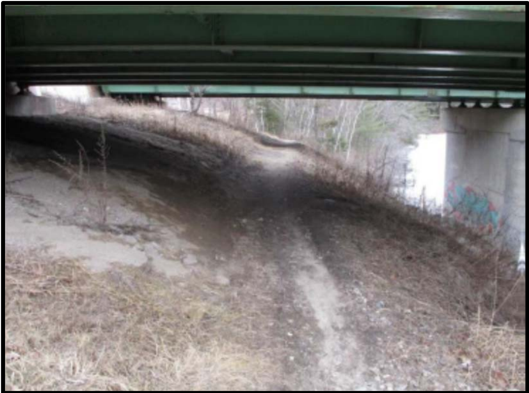
Figure 4 - Footpath at South Abutment
