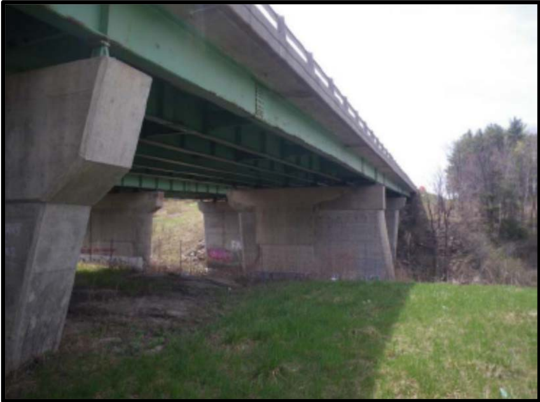
Figure 1 - Southbound Bridge Elevation, Looking South
