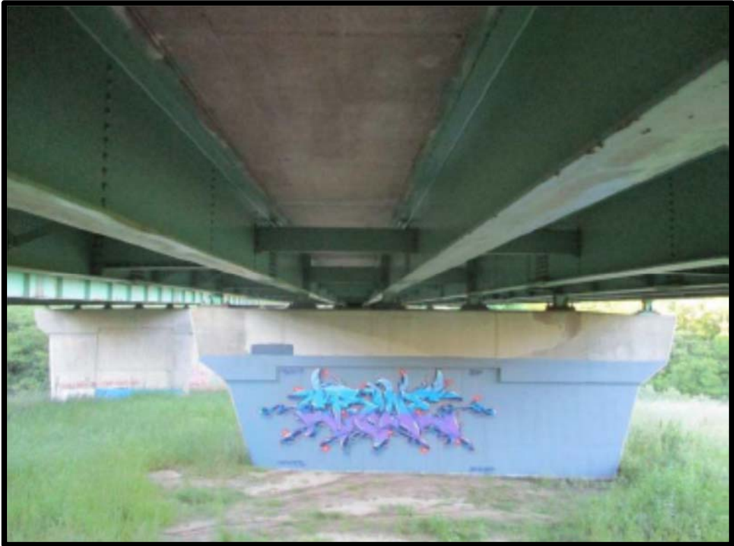
Figure 3 - Southbound Bridge Southern Pier Elevation, Looking South
