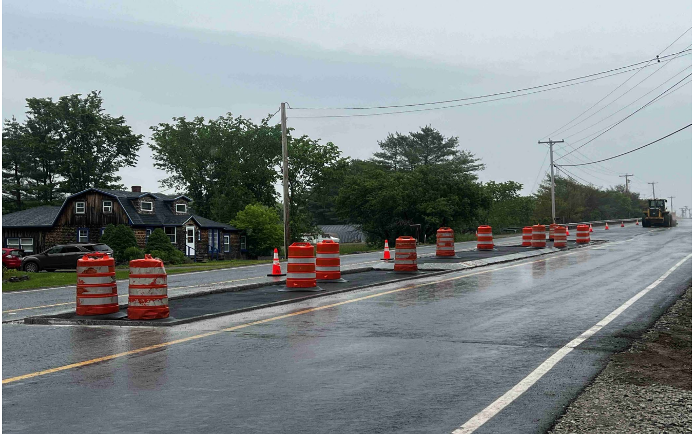
Looking east at one of the new median islands along Route 126.
