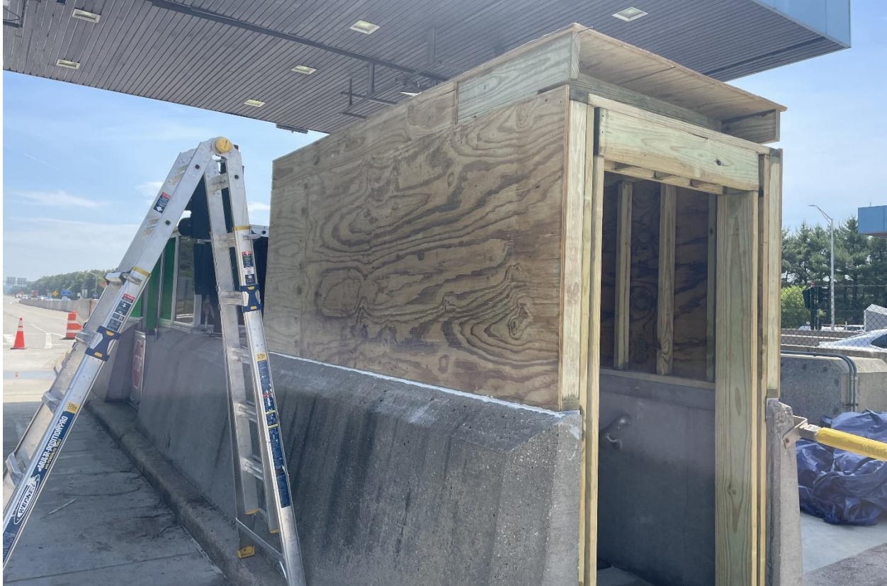
Looking at New Gloucester Toll Plaza northbound stair enclosure for tunnel access.
