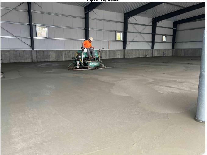
An operator uses a ride on power trowel to finish the concrete slab.
