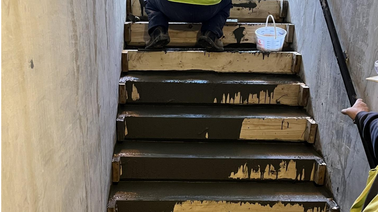
West Gardiner Toll Plaza Southbound Tunnel Stairs resurfacing.
