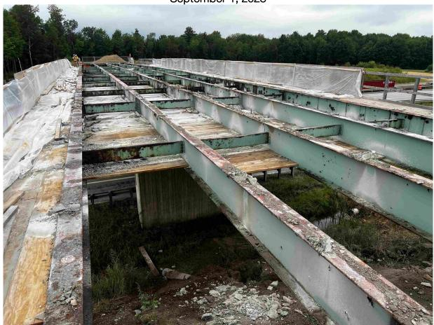
Looking west, the old bridge deck has been removed. The contractor is preparing to remove the existing girders after Labor Day.
