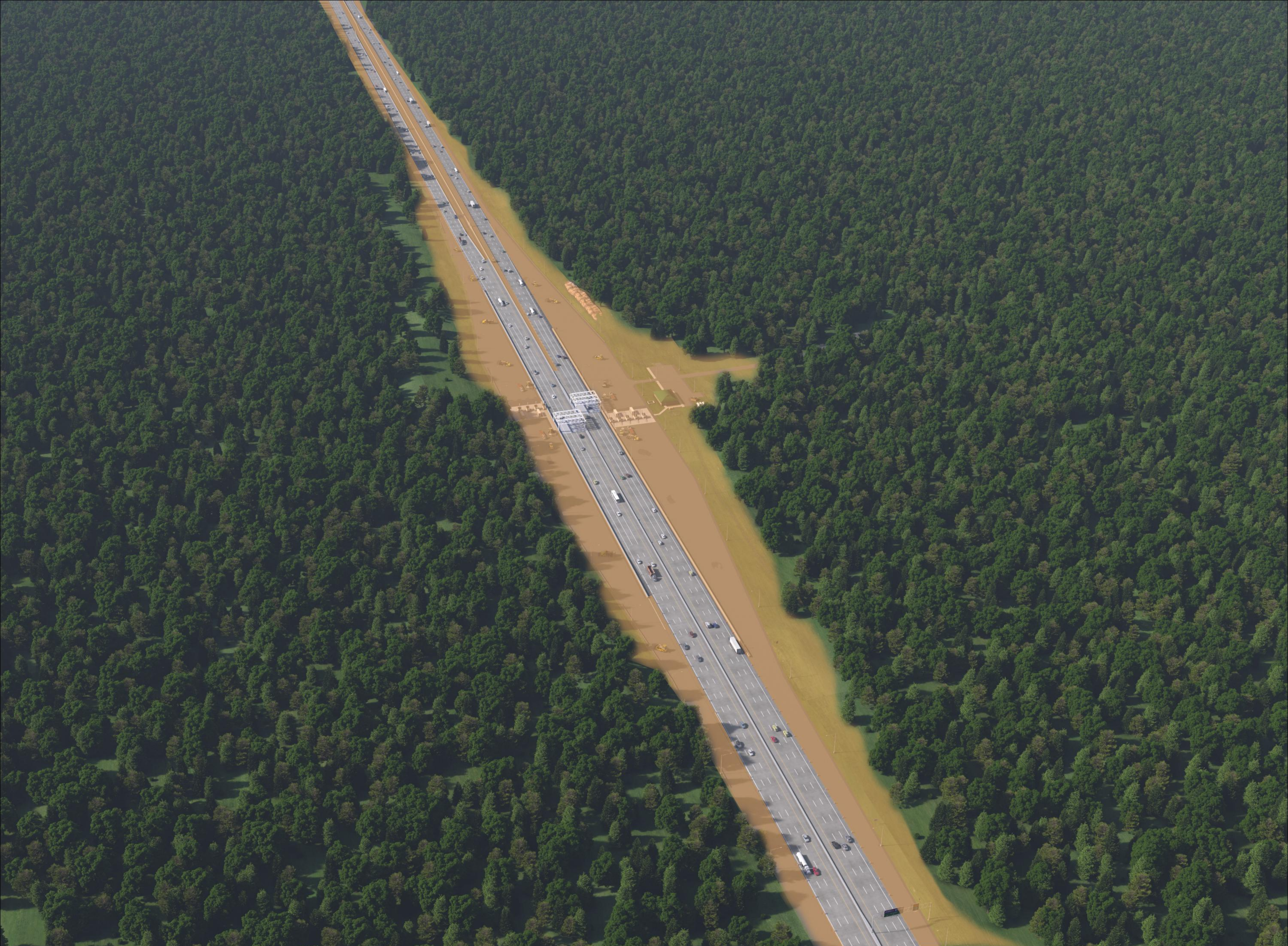
York Toll Plaza at Mile 8.8 - Stage 3
