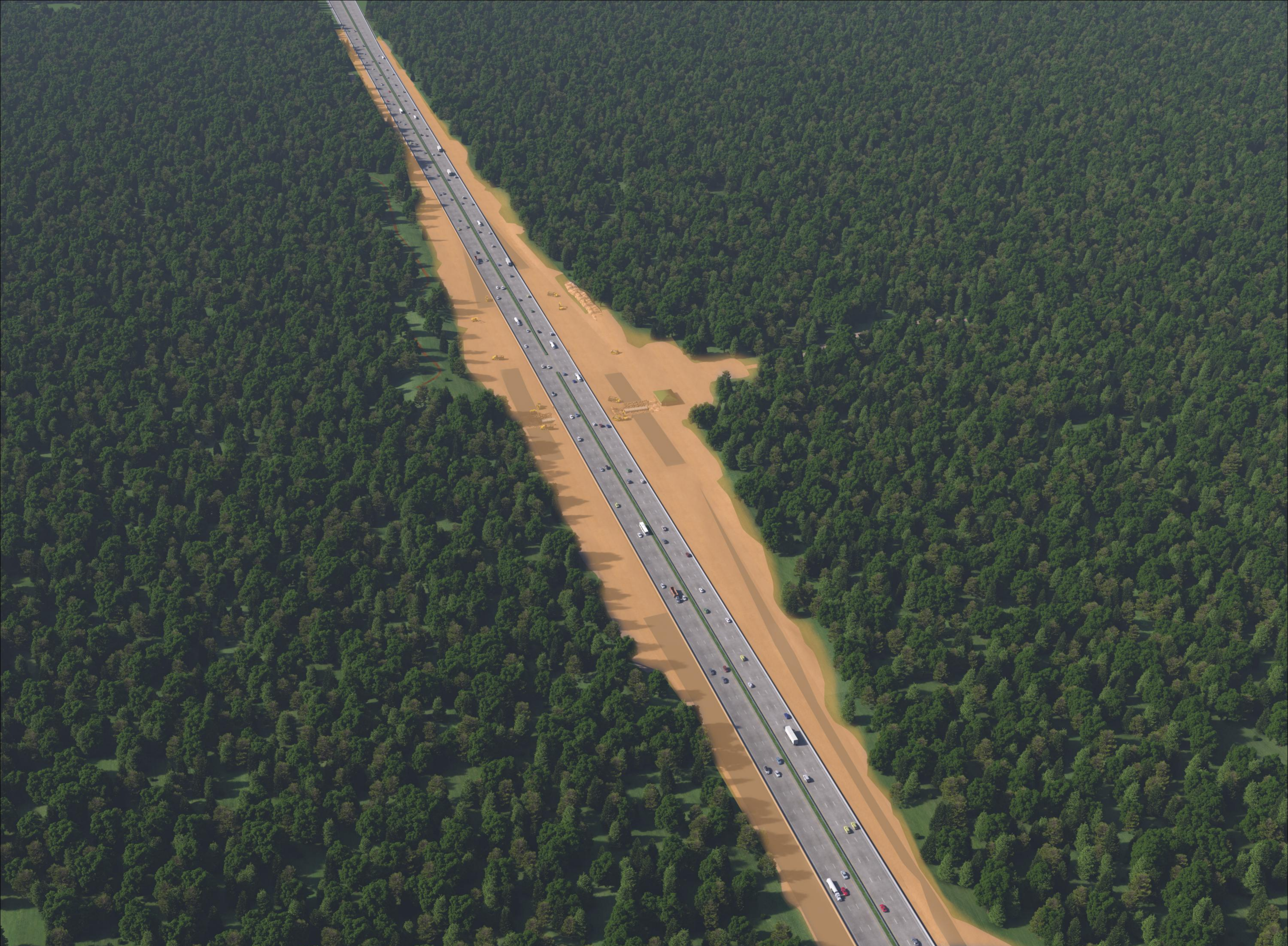
York Toll Plaza at Mile 8.8 - Stage 1
