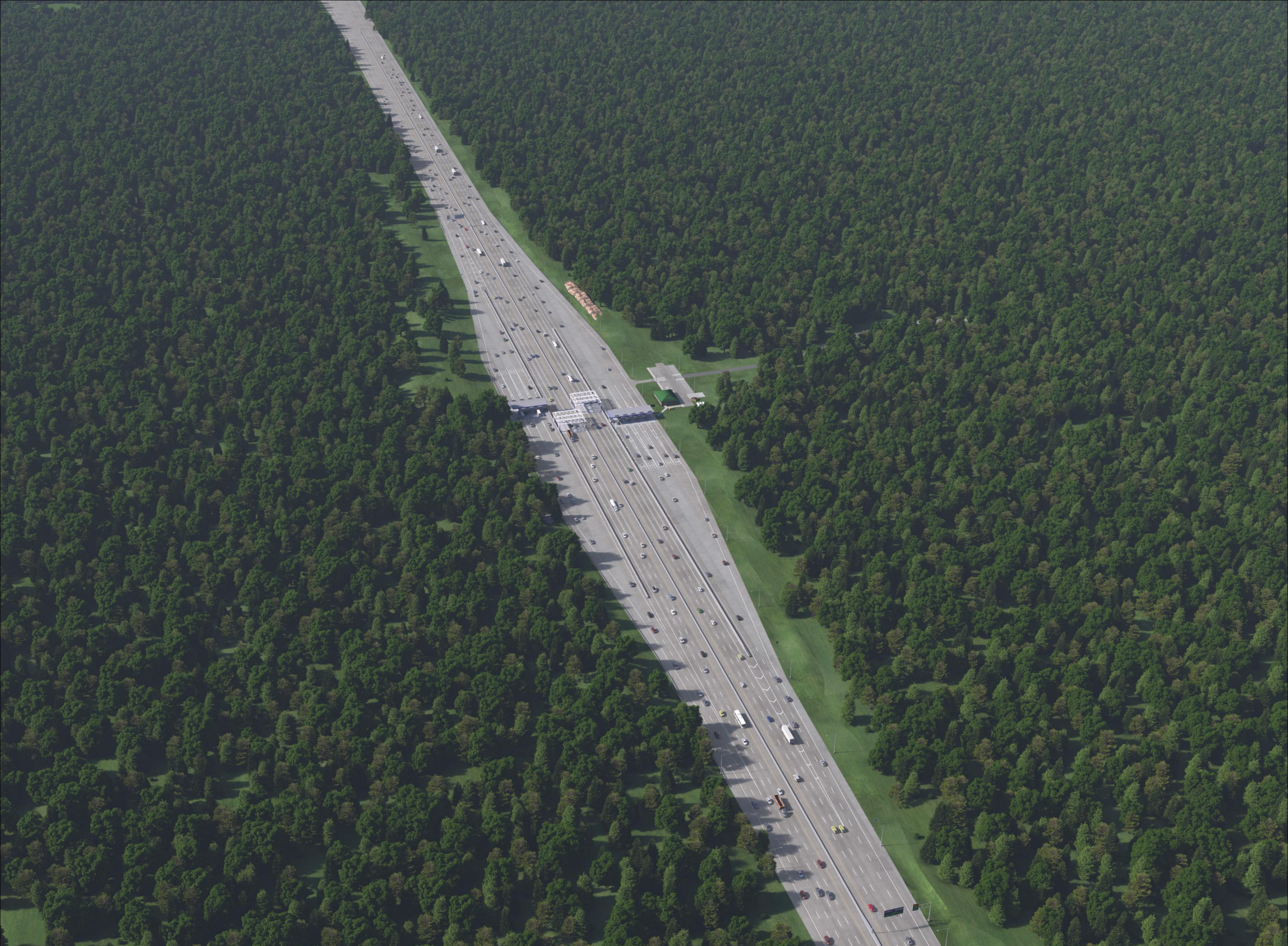
York Toll Plaza at Mile 8.8 - Final Conditions
