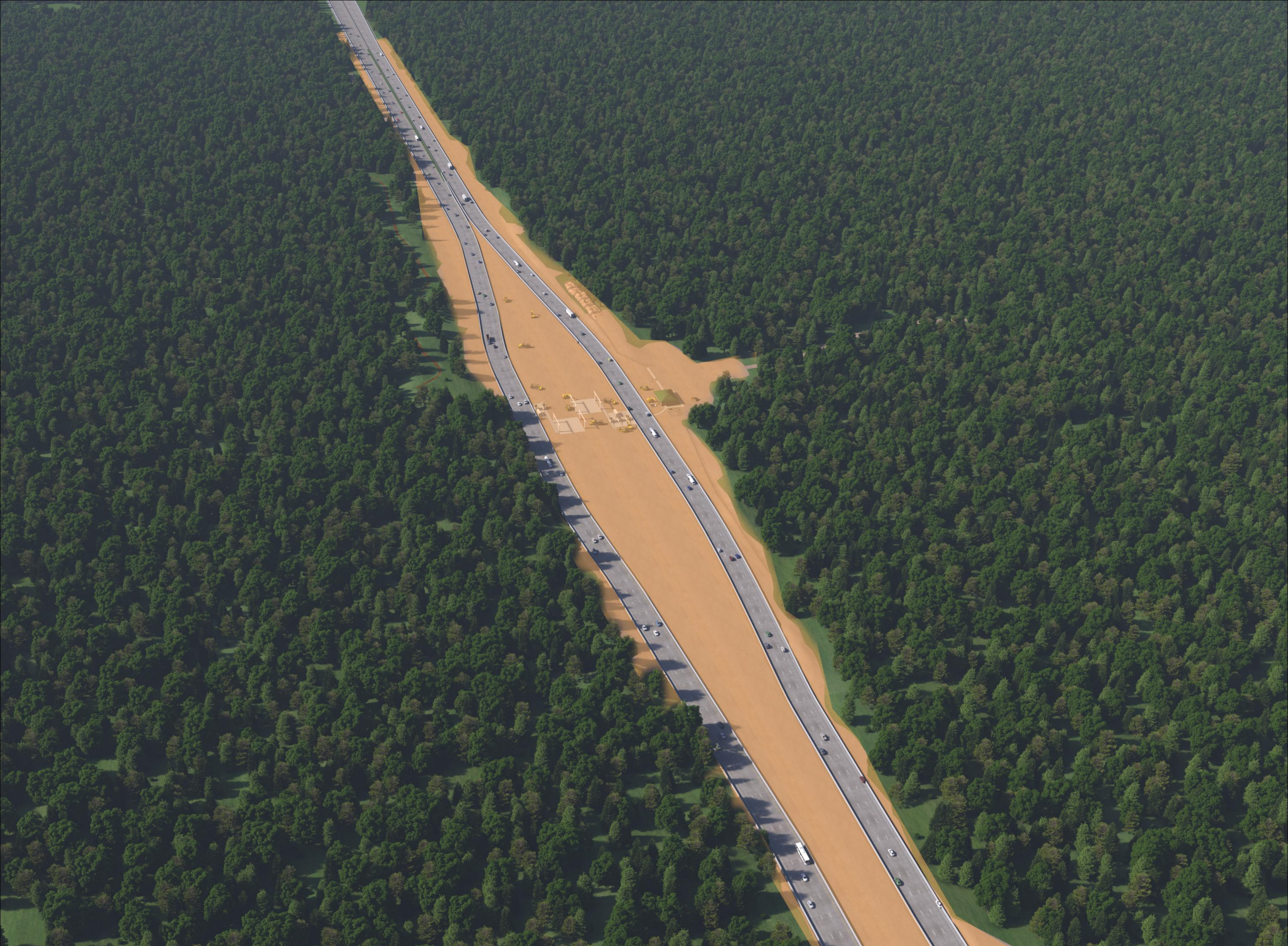
York Toll Plaza at Mile 8.8 - Stage 2
