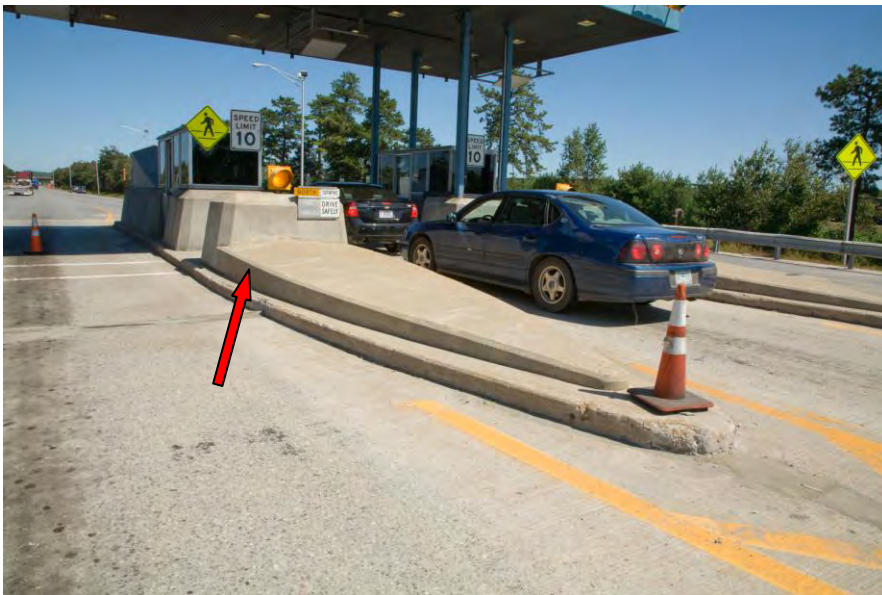
FIGURE 1.6 - New Gloucester Toll Booth, Double Bumper and Raised Median
