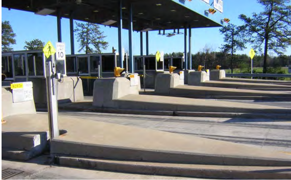
Figure 5 New Gloucester Toll Booth, Double Bumper and Raised Median
