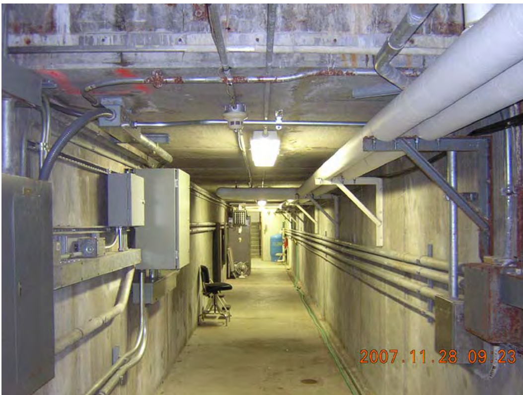
Figure 7 New Gloucester Tunnel
