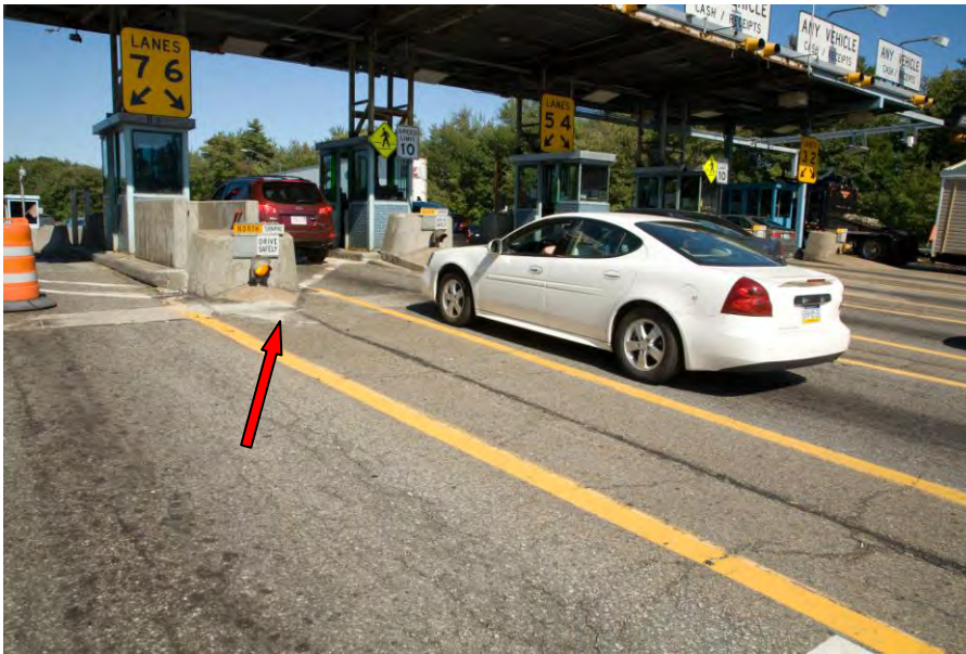
FIGURE 1.5 - York Toll Booth, Single Bumper and Settled Island
