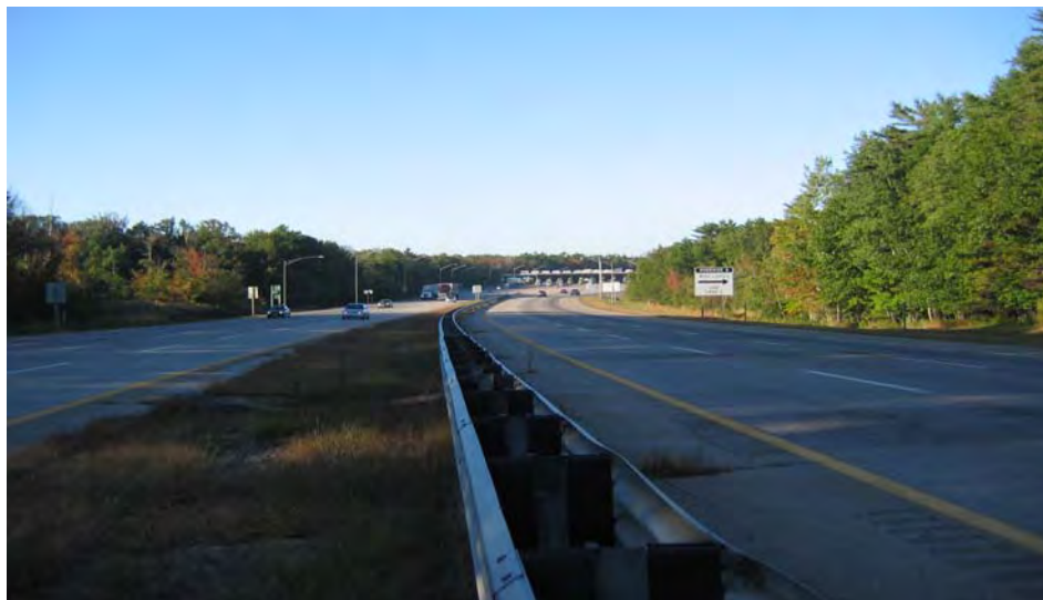
Figure 2 Southbound Sight Distance Horizontal Curve and Down Gradient Are Not Desirable Due To Safety and Operational Concerns
