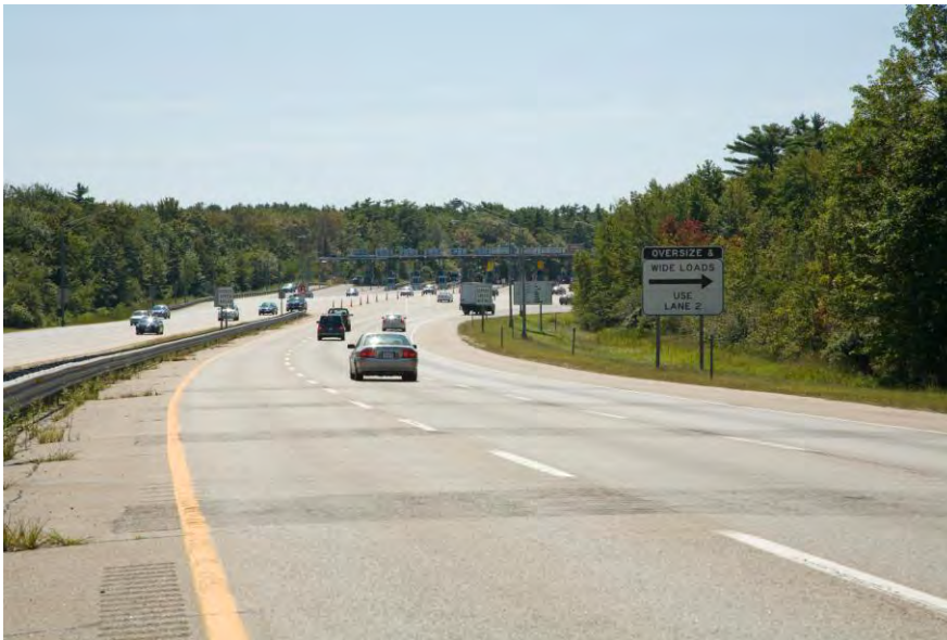
FIGURE 1.3 - Southbound Sight Distance Horizontal curve and down gradient are not desirable due to safety and operational concerns.
