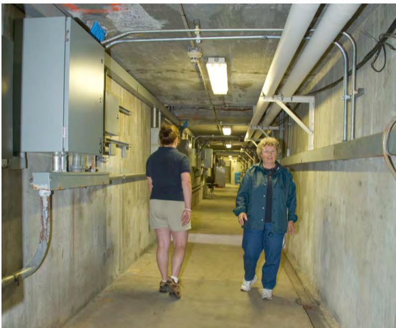
FIGURE 1.10 - New Gloucester Tunnel Note, wide passageway.
