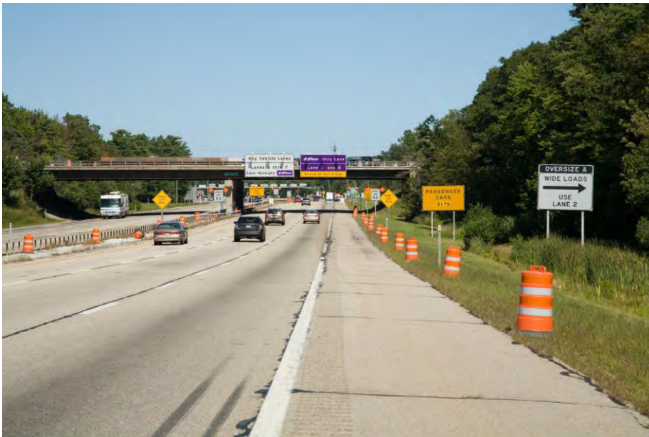
FIGURE 1.2 - Northbound Sight Distance Bridge and horizontal curve negatively impact sight distance.
