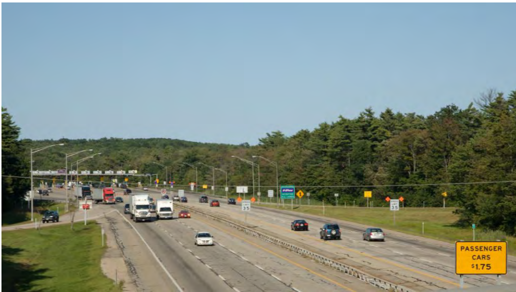
FIGURE 1.1 - Exit 7 Interchange Ramps South of York Toll Plaza
