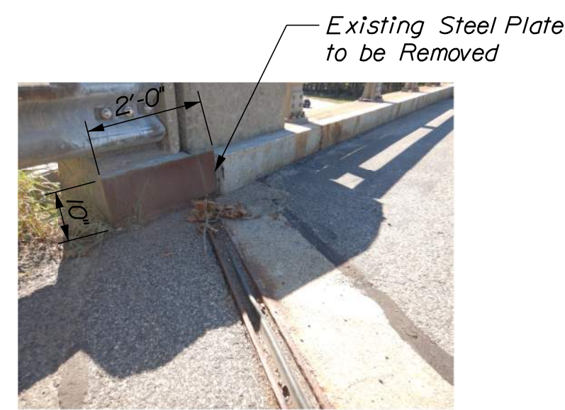
STEEL CURB PLATE ELEVATION Not to Scale
