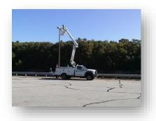
In 2016 approximately 205 existing highway and site lighting luminaires were replaced with LED luminaires at Maine Turnpike entering and existing ramps, toll plazas, service plazas, and maintenance yards. The work included verifying existing luminaire and circuit voltages, furnishing and installing replacement LED luminaires and furnishing and installing pole breakaway splice kits, if non-existent.
