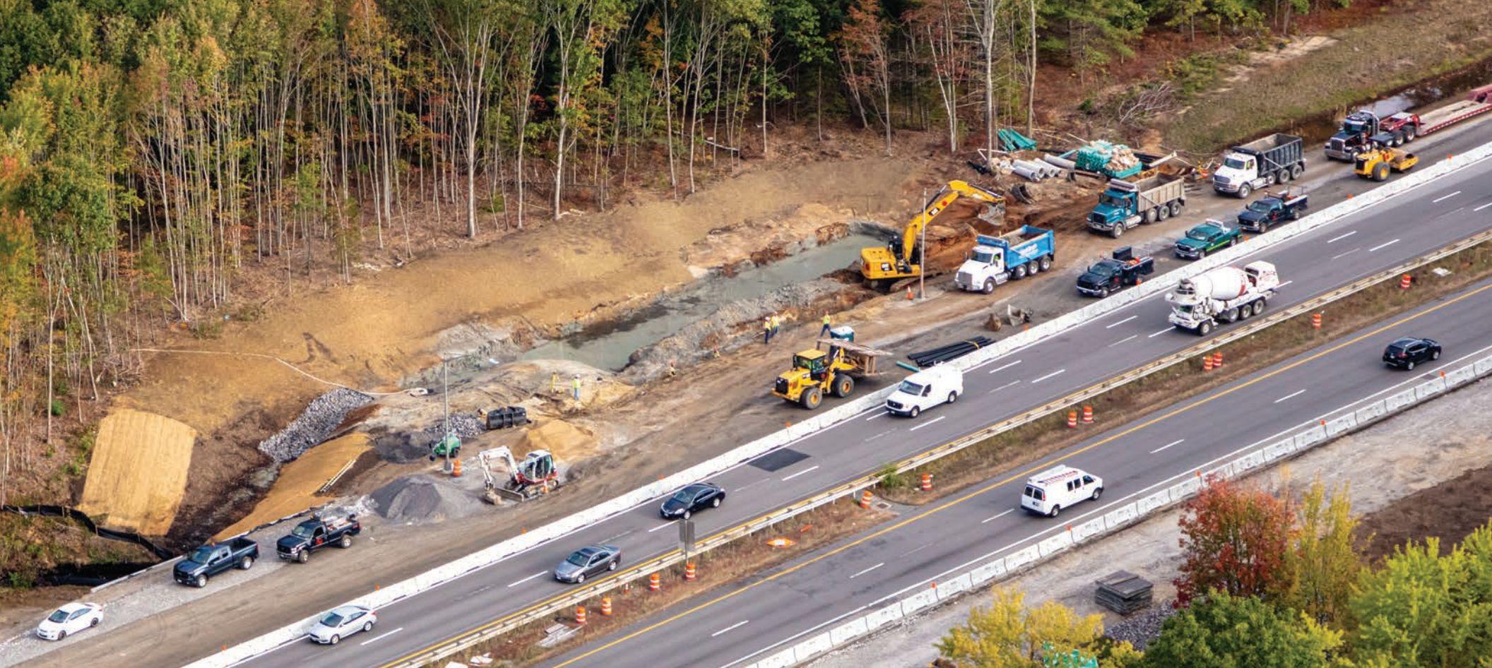
Portland Area Widening earthwork construction at mile 43 in Scarborough
