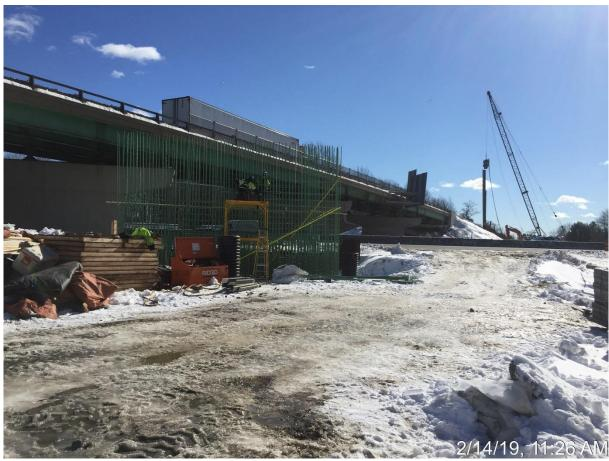
Installing the rebar for the west pier stem, driving temporary earth support system in the background
