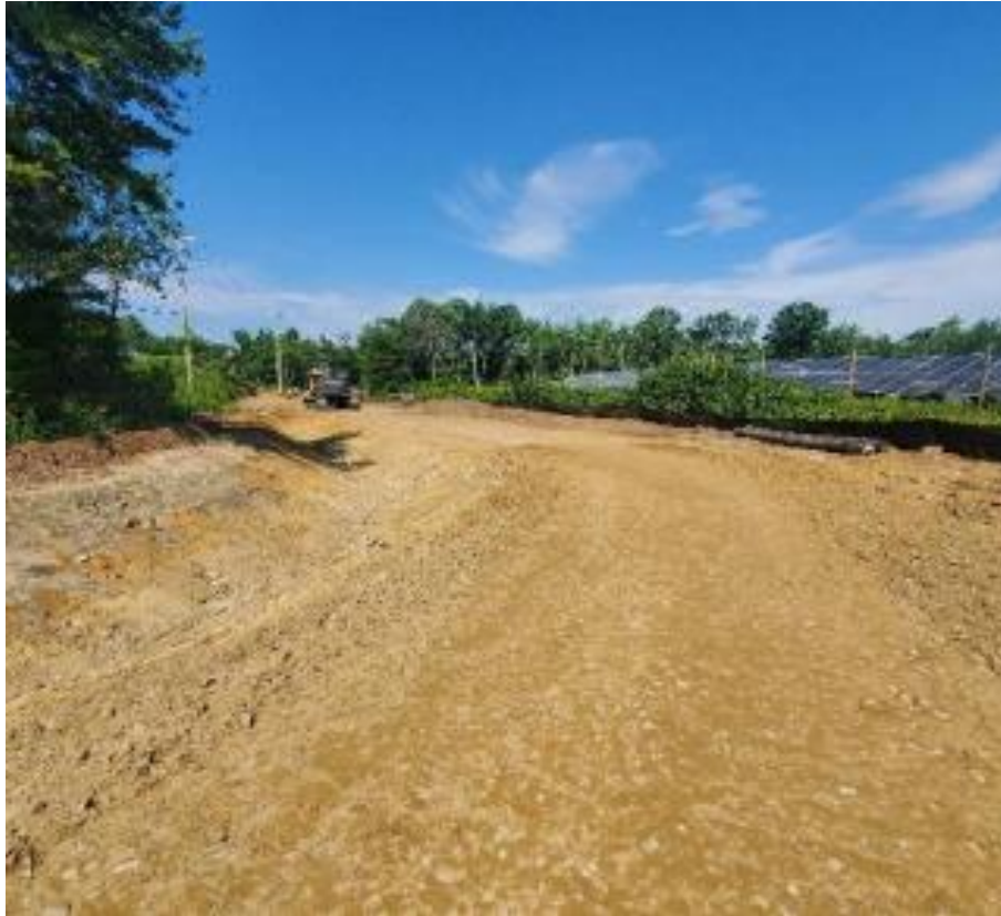
Looking east, crews installing gravel on Northbound Emergency Vehicle Ramp
