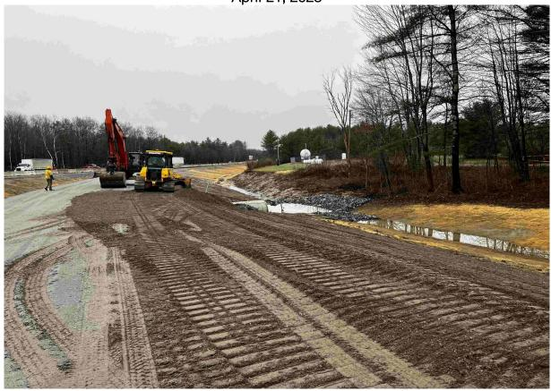
Looking south down the new ramp, Grondin crews are shimming with Type D gravel.
