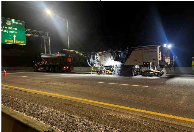
Heading west on the 703, a milling crew profiles the existing pavement to match modern highway standards. Improve drainage, and ride quality.
