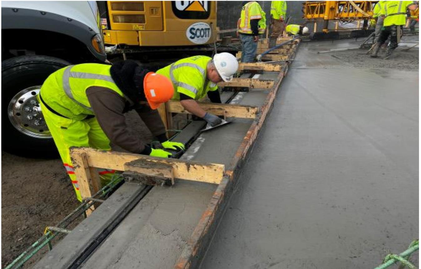
Scott Construction crews are hand-finishing concrete at the eastern bridge abutment joint.
