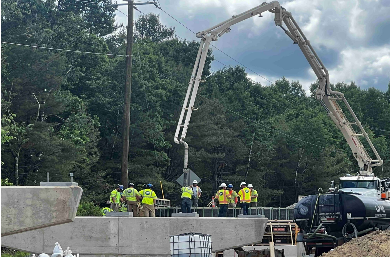
CPM Crews are placing concrete in the East side abutment.
