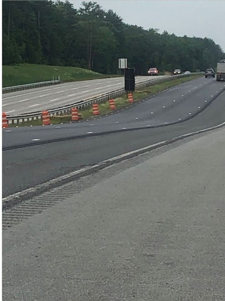
Looking south bound, near MM 40.0.
