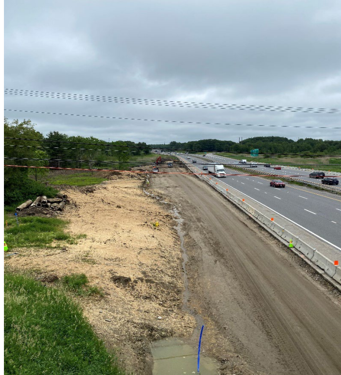
Collector distributor road looking northbound.
