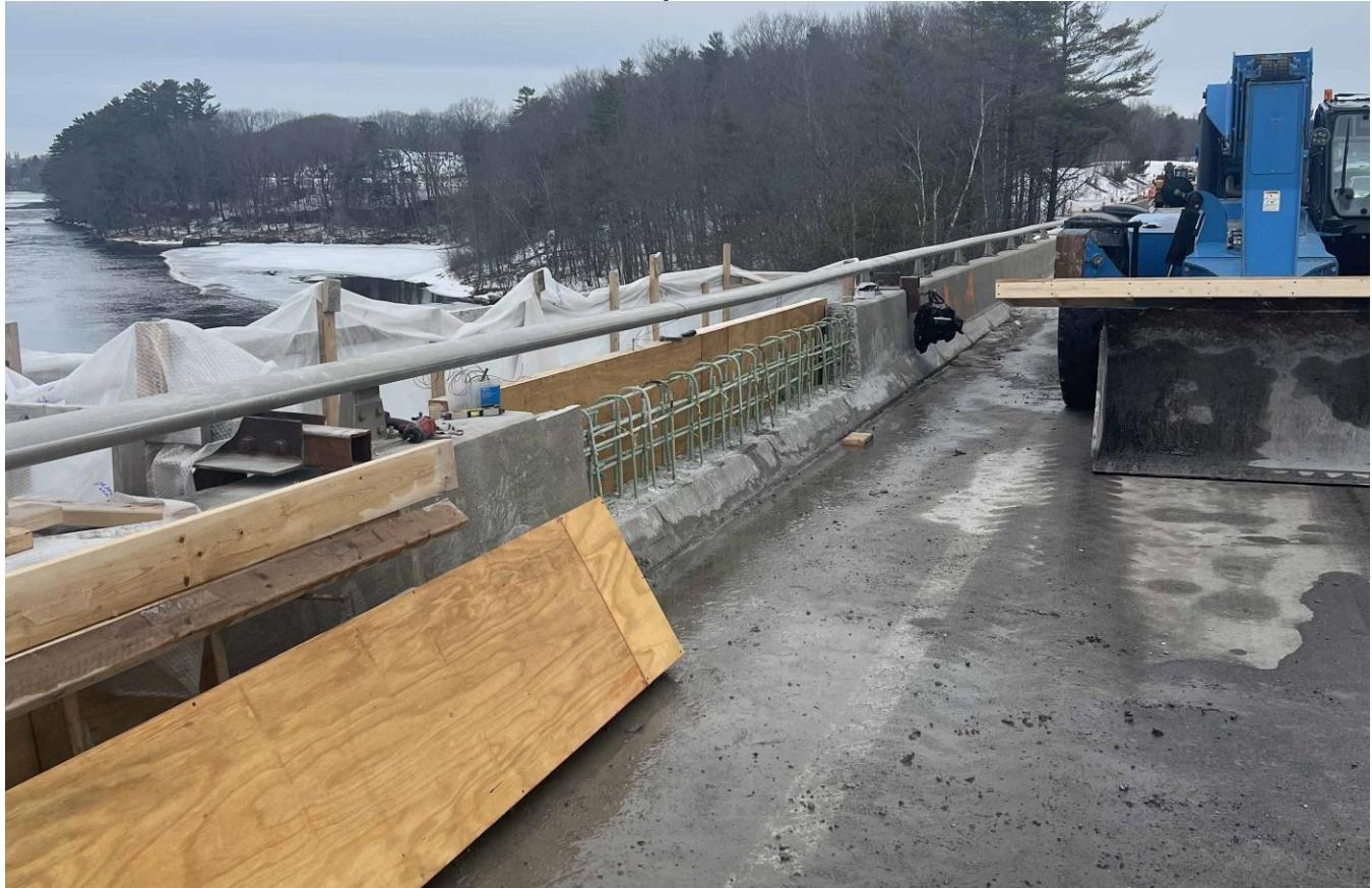
Looking at the Southbound parapet with formwork in place waiting for warmer weather
