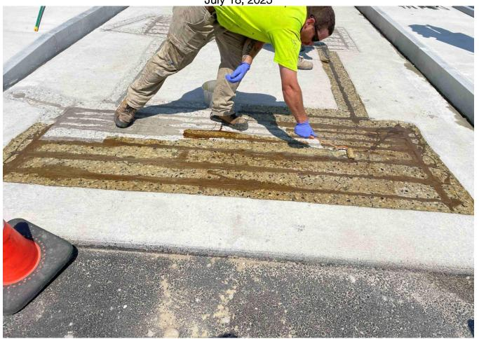
Laborer rolls out epoxy over the recently installed toll loop.
