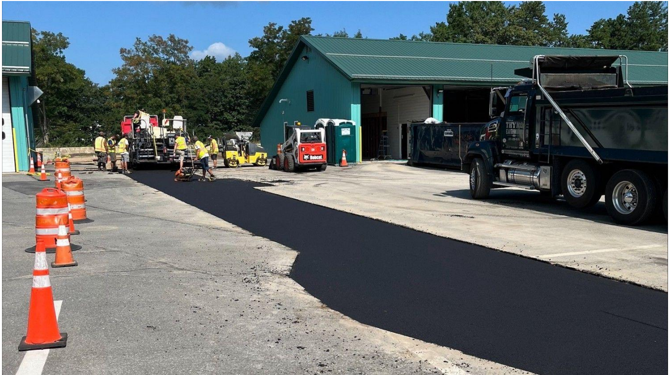
The contractor paves the water main trench.
