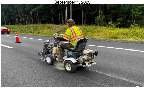
At the beginning of the northbound lanes, the recessed grooves for the reflective tape are being ground with a powered milling machine.
