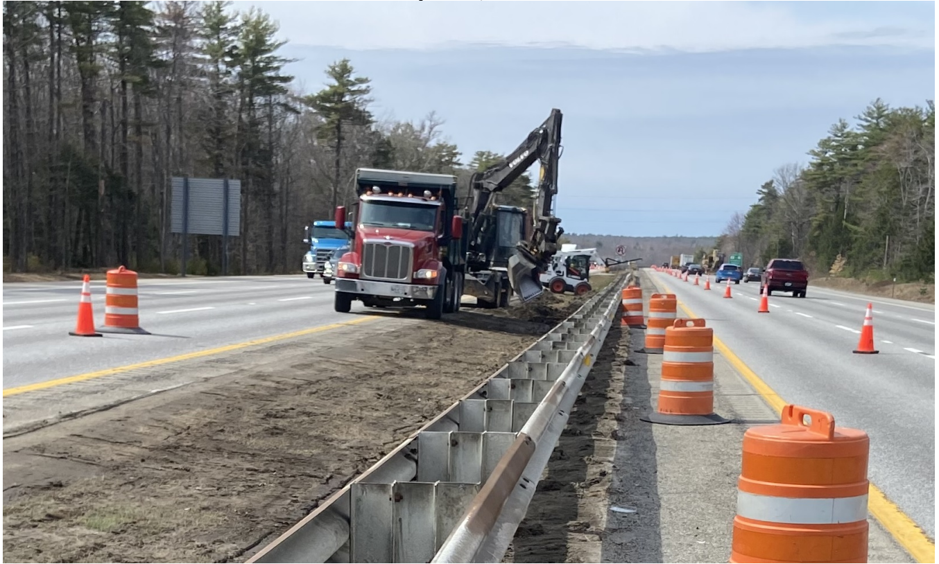
A Grondin crew regrades the median at approximately MM33, looking south.
