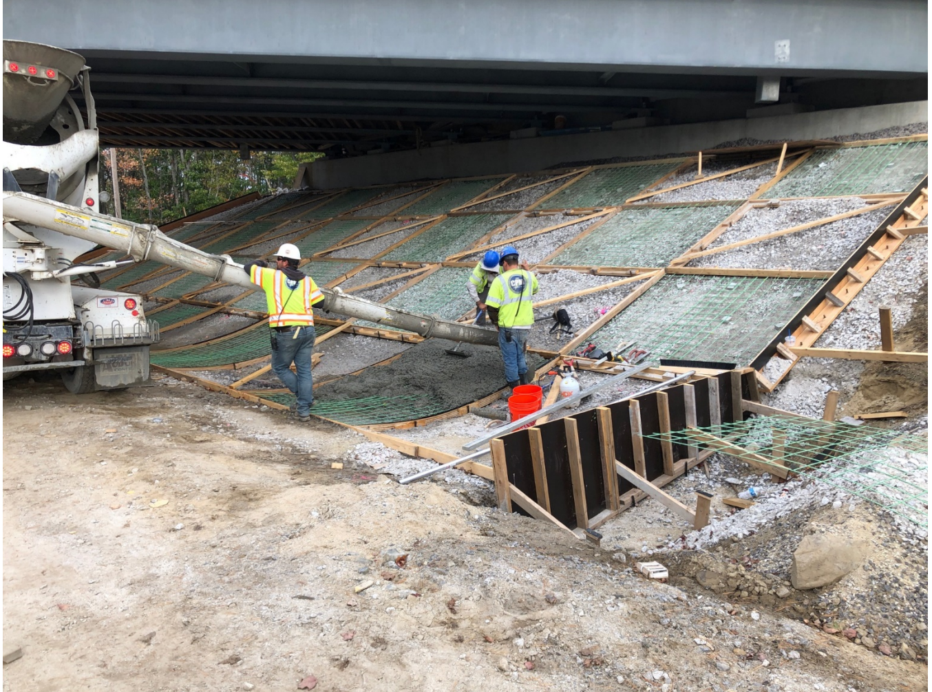
Concrete slope protection
