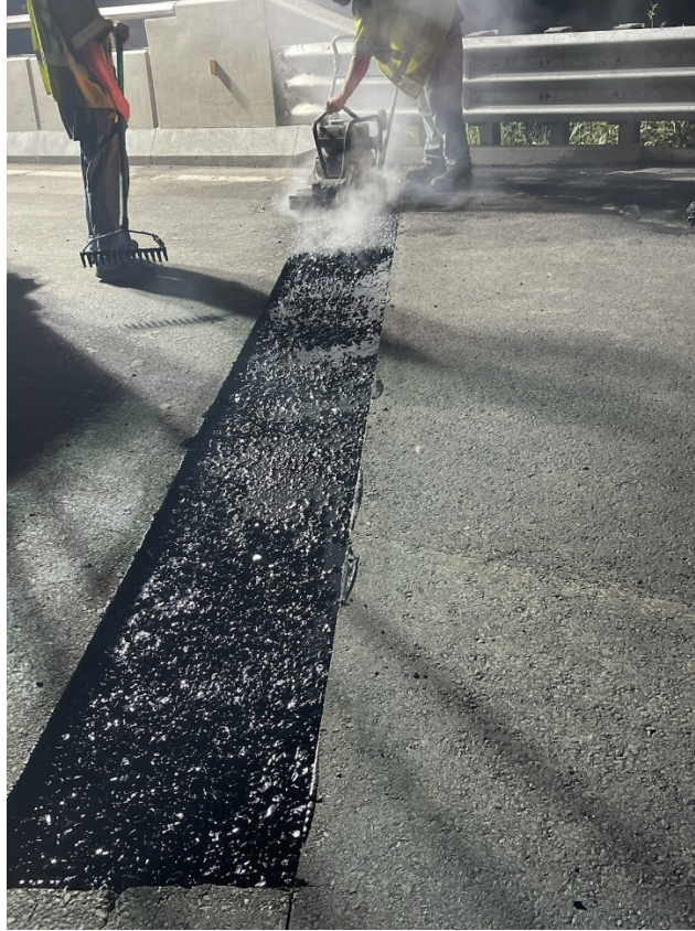
Installing Asphaltic Plug Joint
