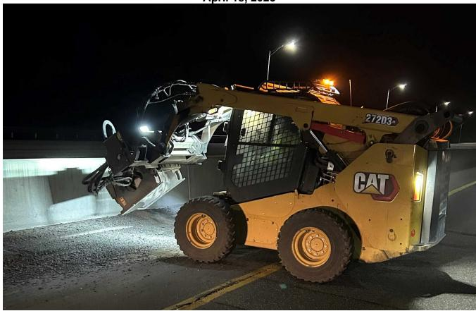
Contractor uses a skid steer to grind around the storm drains before paving
