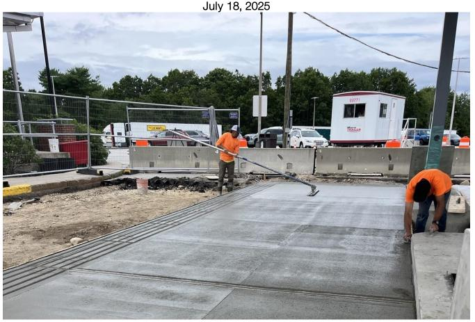
The concrete finishers are floating the slabs at the rehabilitated gas dispensers.
