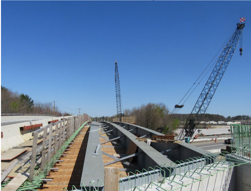
Looking west at phase 2 girders
