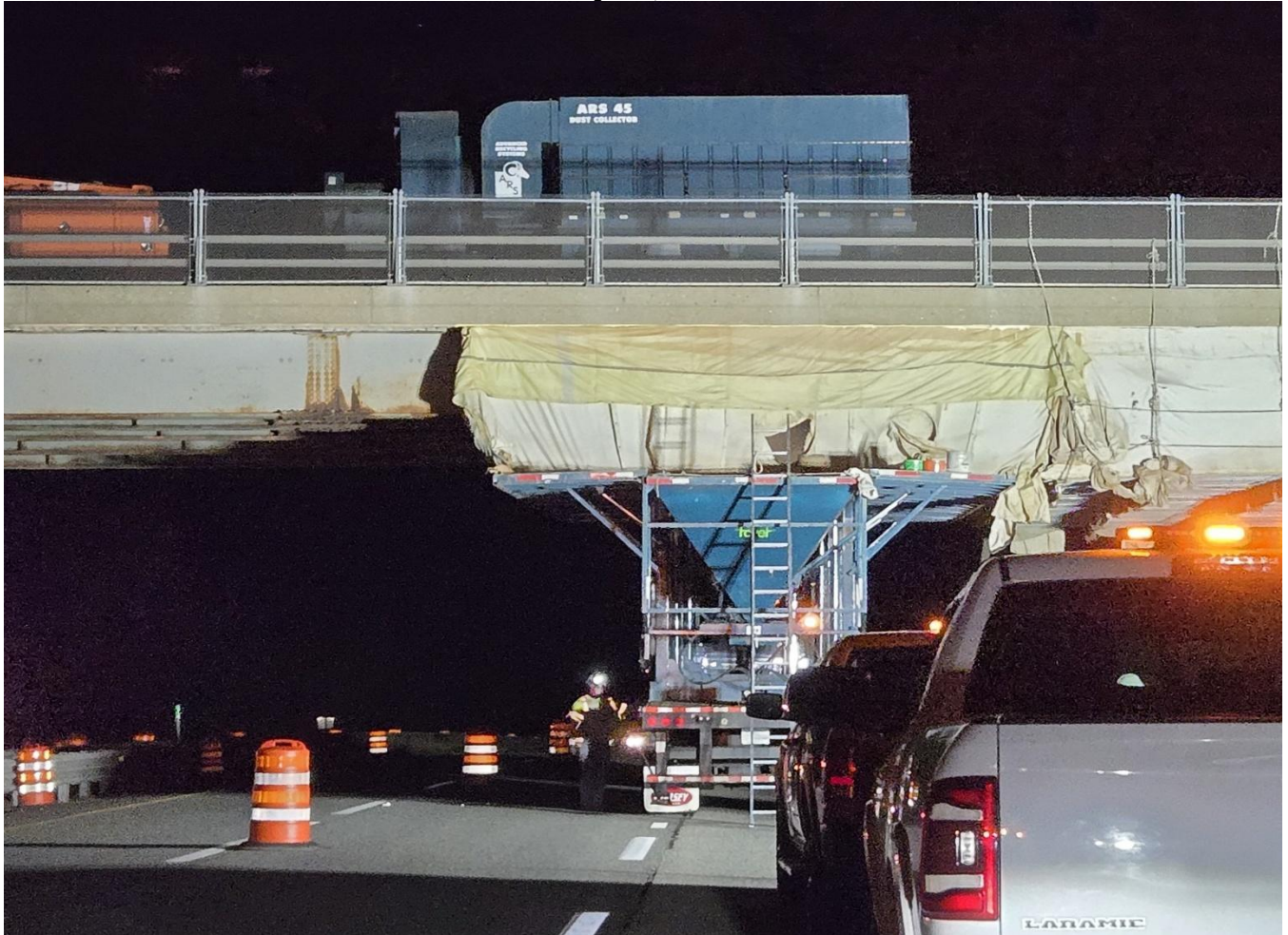
Mountain Road (York), looking north at the media blasting operation.
