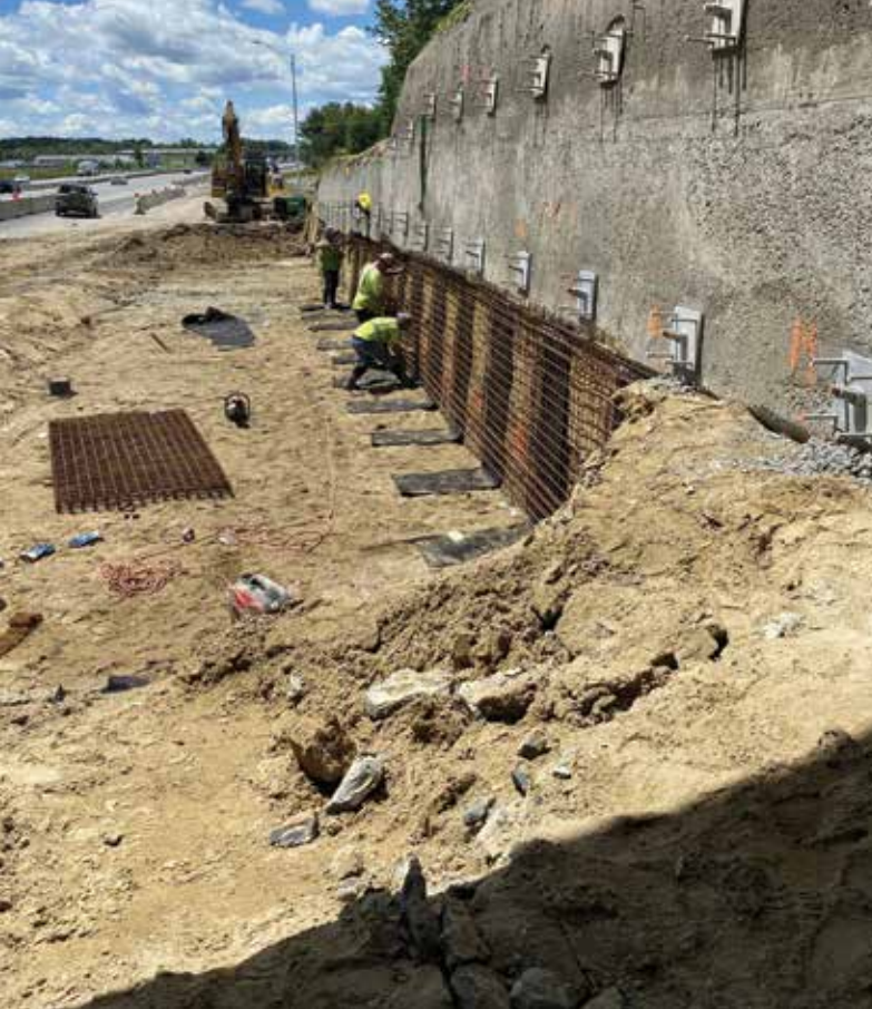
Crew place reinforced steel as part of a new soil nail wall
