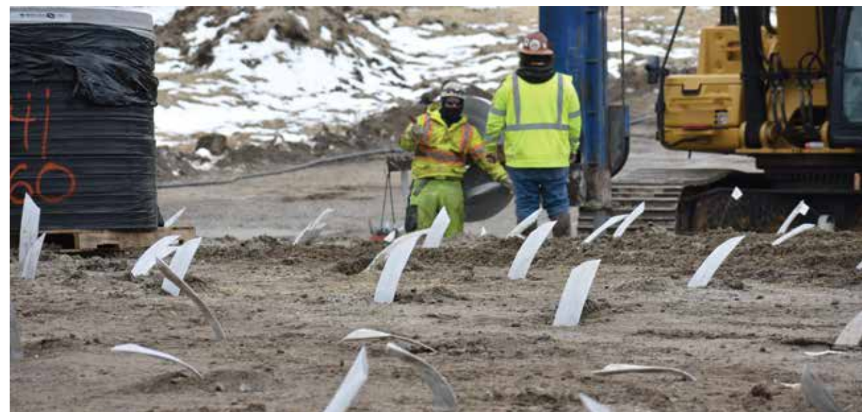
Wick drains installed to prepare the ground for the future toll plaza
