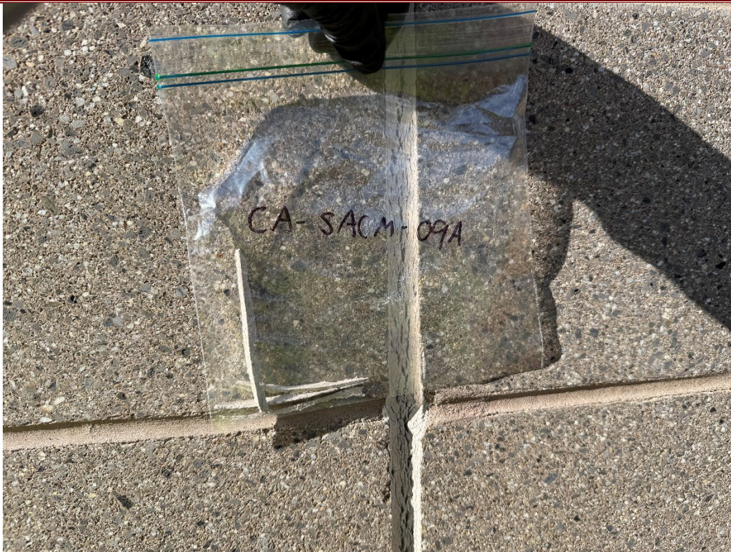
9. View of CA-SACM-09, expansion joint caulk, gray
