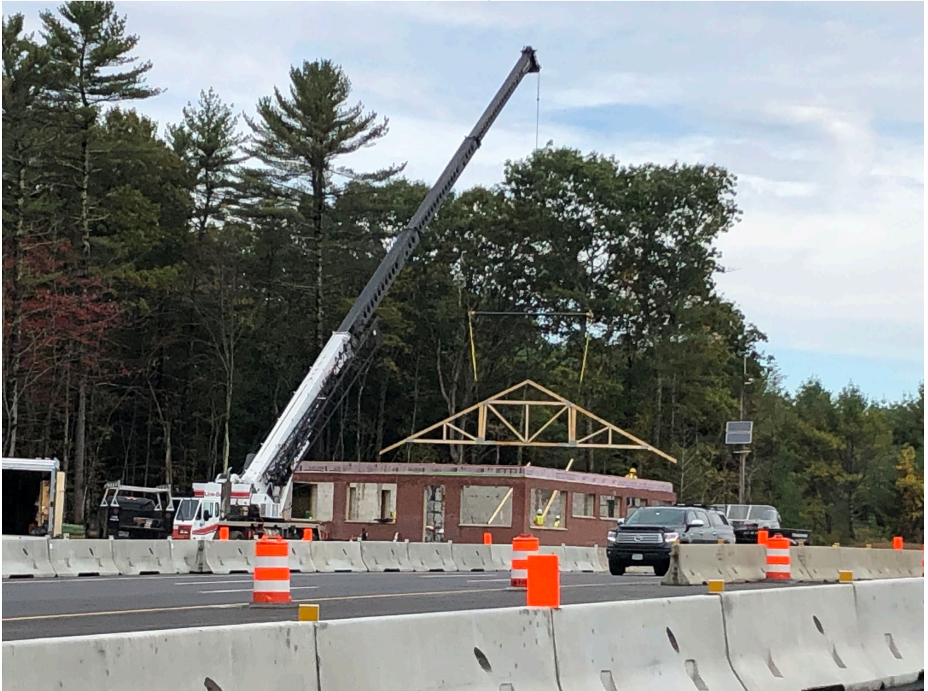
Contractor setting the first truss of the toll building.
