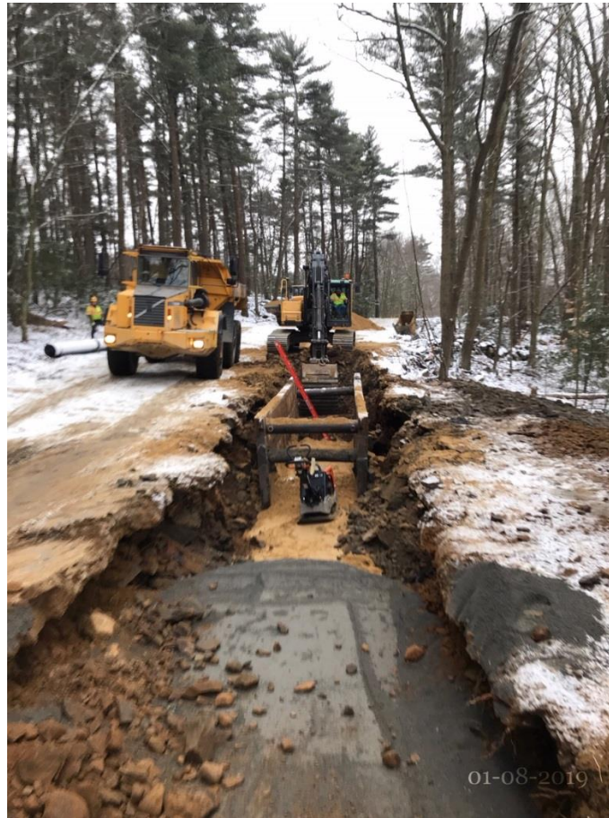
Installing waterline
