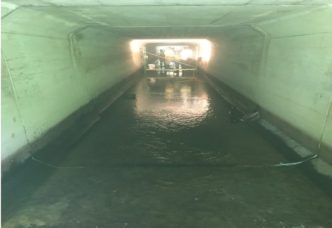
Inlet side of the Thacher Brook culvert.
