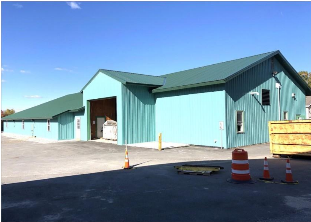
Photo 2 – Building rear elevation
