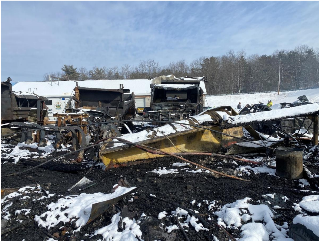
Photo 9 – Building remnants, including equipment
