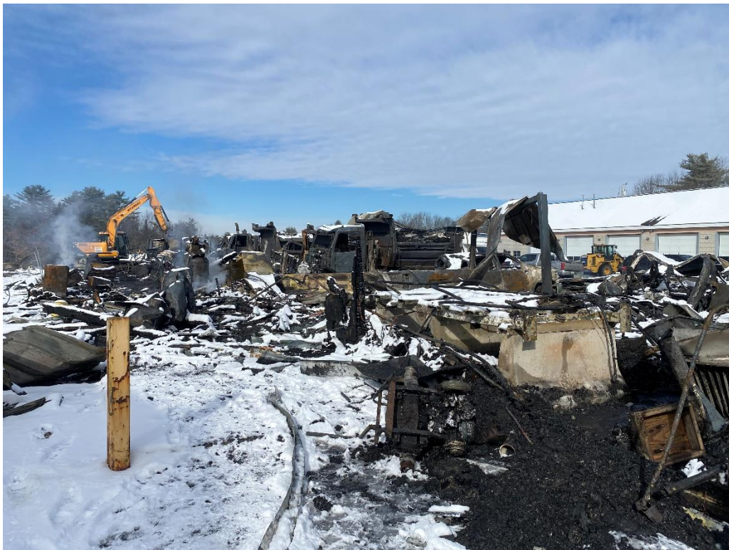
Photo 4 – Building remnants, including equipment
