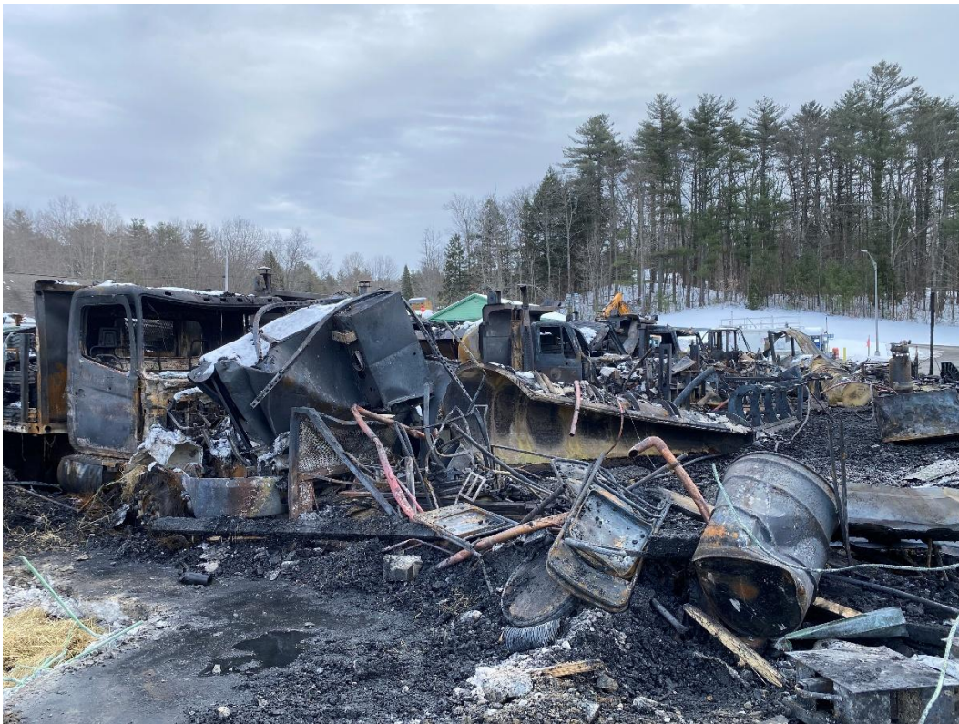
Photo 7 – Building remnants, including equipment
