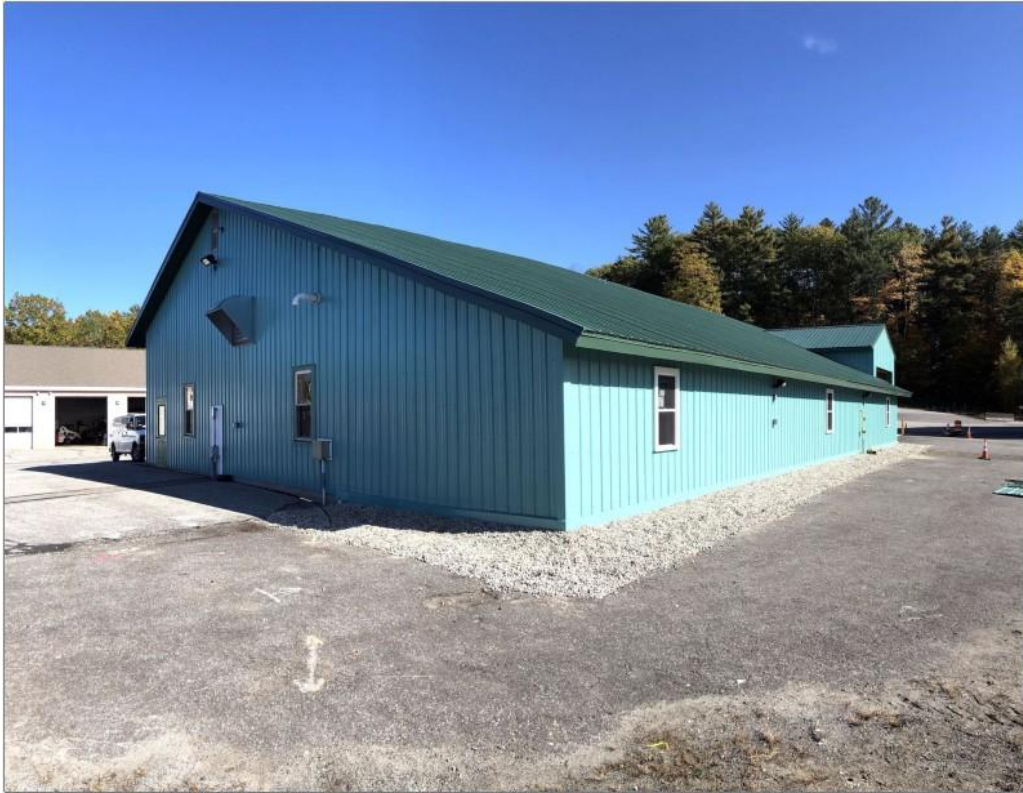
Photo 1 – Building side elevation
