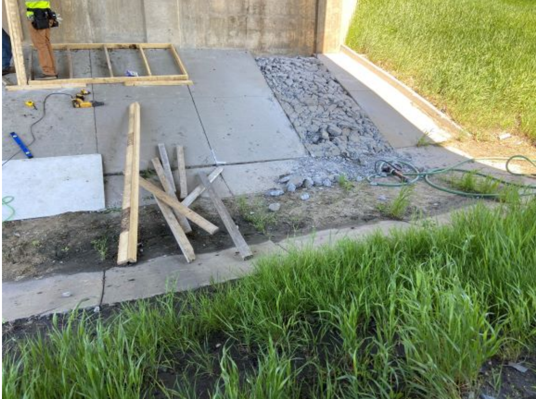
Boom Road south bound abutment slope protection panel repairs.
