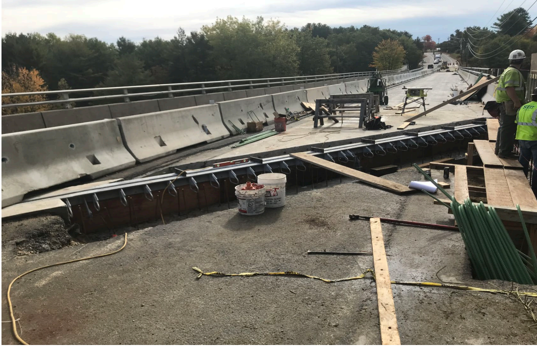
Shaker Road Bridge new joint installation in progress.
