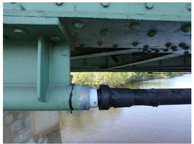
**Figure 1 – Failed Anchor Block Sleeve**
