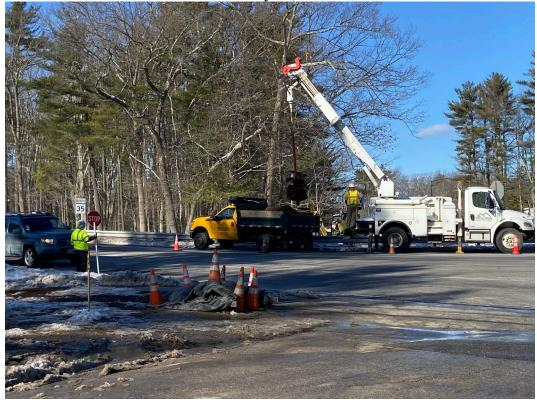
Crews excavate for the one of the mast arm foundations at the intersection of Fletcher St and the NB Exit 25 Ramp.
