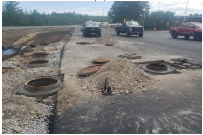
Access covers to the oil water separator being installed at the NB plaza.
